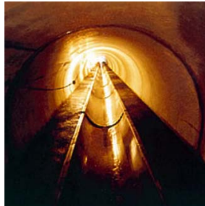
Heat from wastewater – The new energy source
