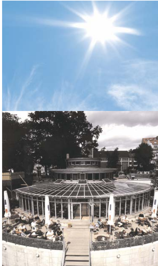
Photovoltaik Cafe Ambiente
