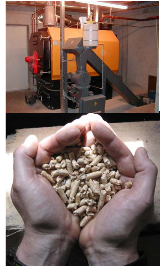
Woodpellet heating system Bavendamm
