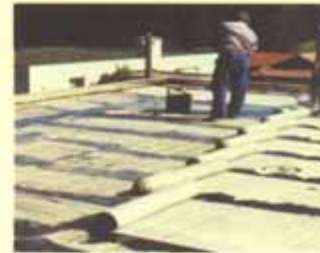
Roof: Installation of single-ply waterproofing membrane
