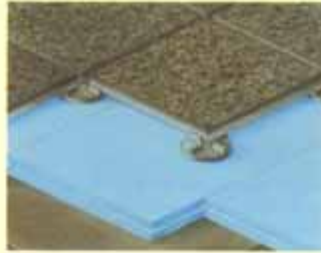
Roof pavers on spacers over Roofmate ®
