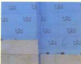
Insulation behind marble
